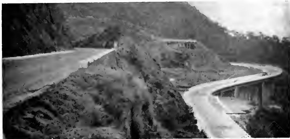
Escarpment section of divided express highway from Santos to Sao Paulo in Brazil
